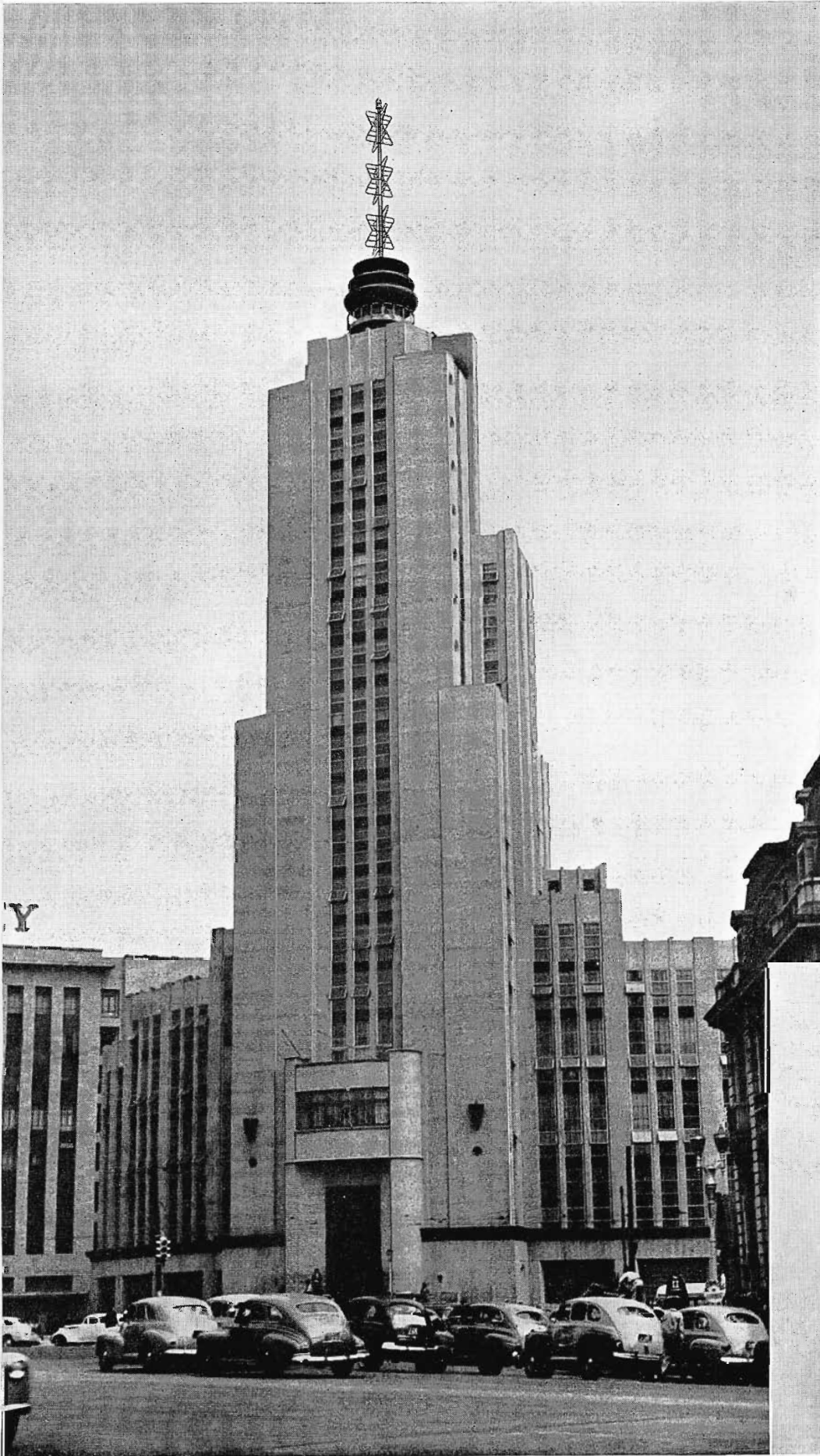
FIG. 10 (above). View of XHTV's three-section Super Turnstile Antenna which is located atop the National Lottery Building.
