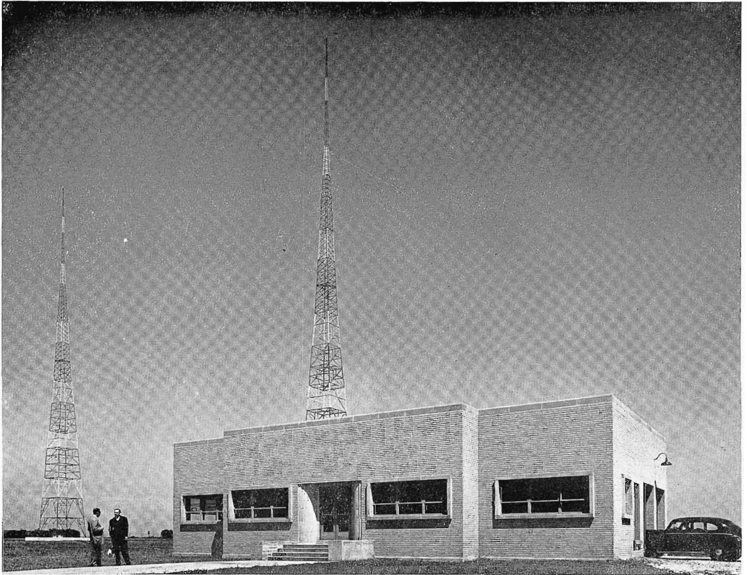
FIG. 10 (above). KSD's AM transmitter at East St. Louis is housed in this brick and stone structure, where all the facilities required for maintenance of equipment and convenience of personnel have been provided. Two towers of the four-tower KSD antenna array are shown in the background.
