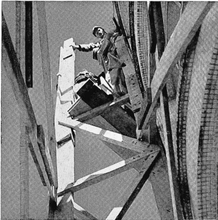
FIG. 20 (above). View of wooden superstructure constructed at top of the Sao Paulo State Bank Building during antenna installation.
