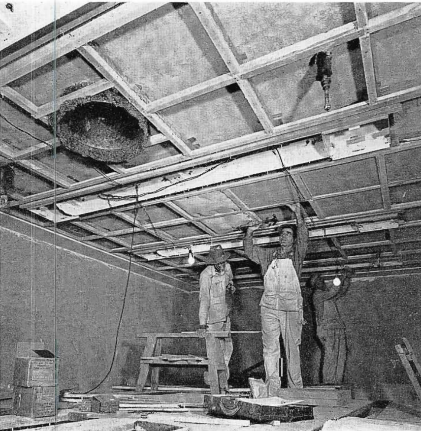
FIG. 8. The studio ceiling is completely surfaced with perforated transite over special acoustical material. Air-conditioning outlets and fluorescent fixtures are flush mounted.
