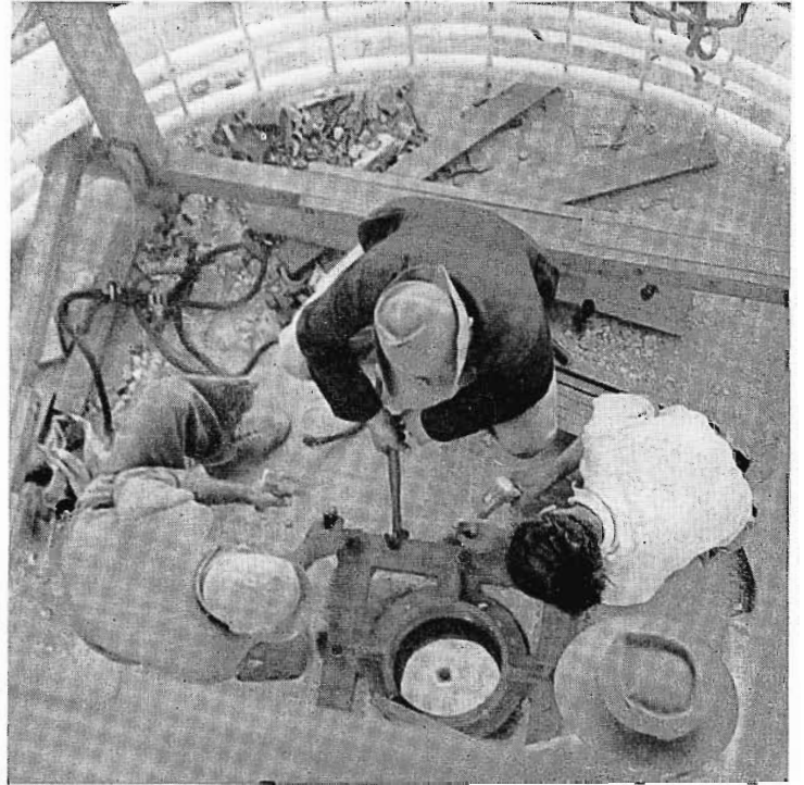
FIG. 21 (above). In this view workmen are shown constructing a suitable base for "seating" the tower.
