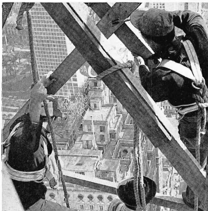
FIG. 22 (below). In this view riggers are shown attaching cables preparatory to lifting the television antenna from the ground floor.
