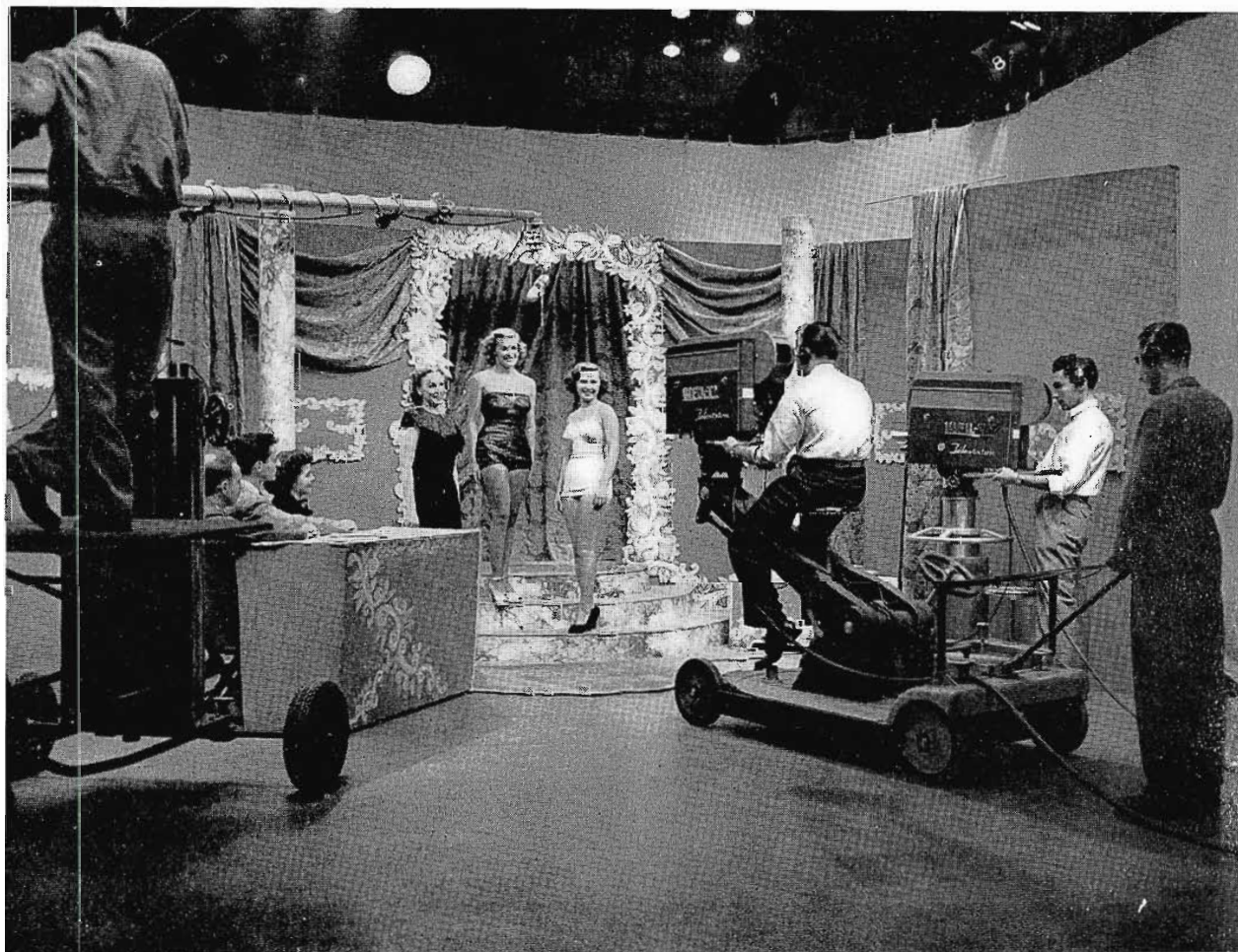
FIG. 8. Another studio setup (courtesy of WFIL-TV) which shows how the RCA boom and microphone arrangement can be used to accommodate a small stage group, yet allowing them sufficient freedom of action.
